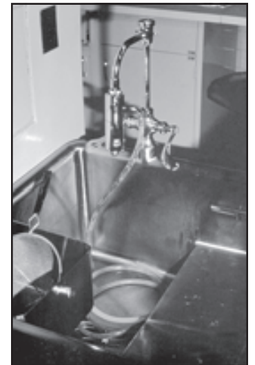
FIGURE 17. Atmospheric vacuum breaker in plumbing supply system.
