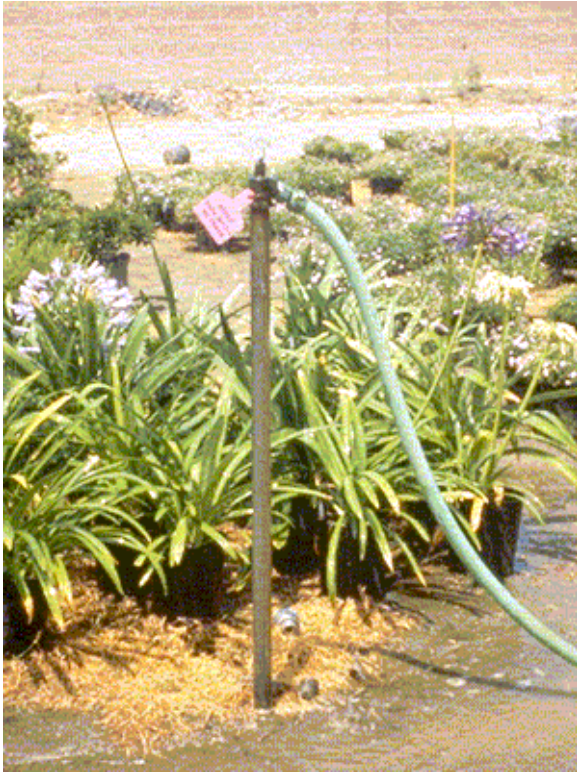
Hose bibbs may only be used with recycled water in areas where they cannot be accessed by the general public (such as this commercial nursery), and even those must be properly labeled.
