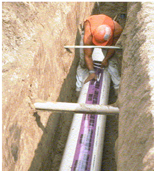
Recycled water pipeline installation with continuous purple warning tape.
